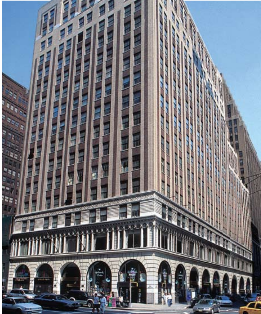
501 Seventh Ave., among the first of the W&H portfolio to receive a makeover, won back-to-back BOMA/NY Pinnacle Awards: first as best renovated building, and as best managed building in its size class a year later.
